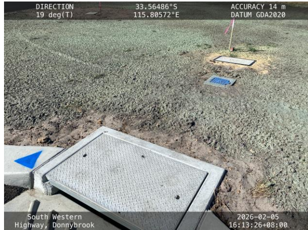
Photo 4 - Fire Hydrant with verge marking
